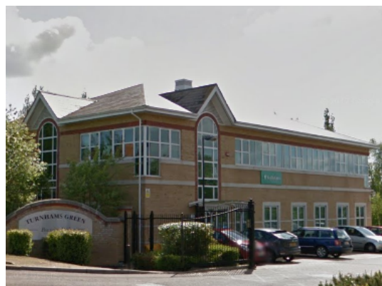
Turnhams Green offices
